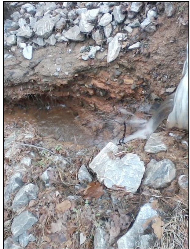
The channel in the dam is over 8' deep now
